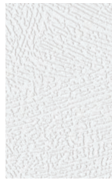
L01 Plaster wall
